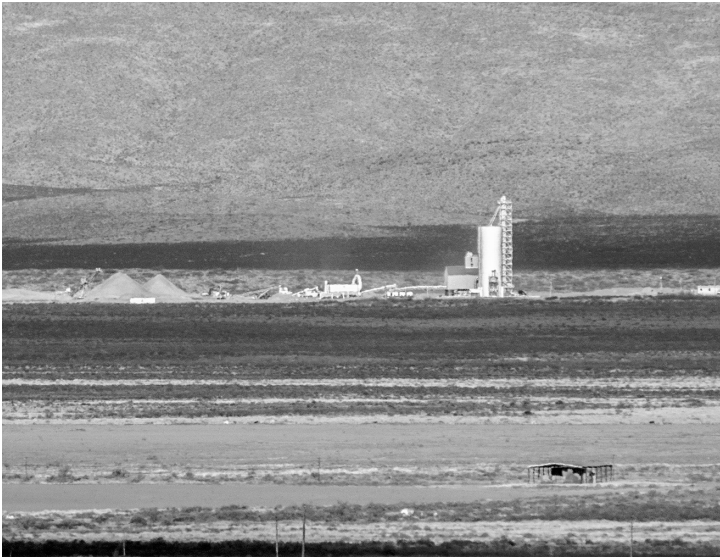
Blue Origin suborbital launch facility, West Texas. Photograph by Kate Crawford
